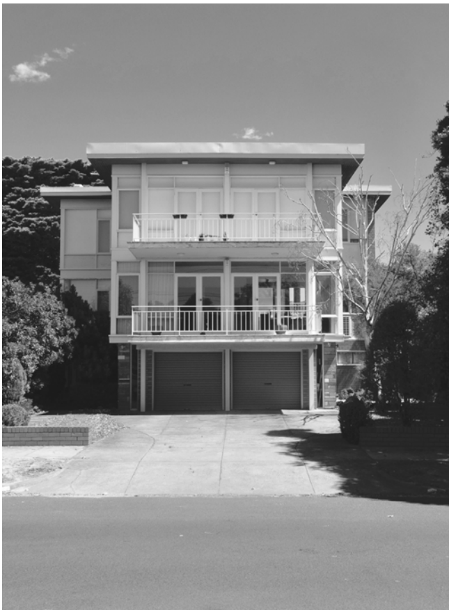
Kluska flats, 1963, 55 Wanda Rd Caulfield North, Ernest Fooks. Photograph: Theo Blankley.
