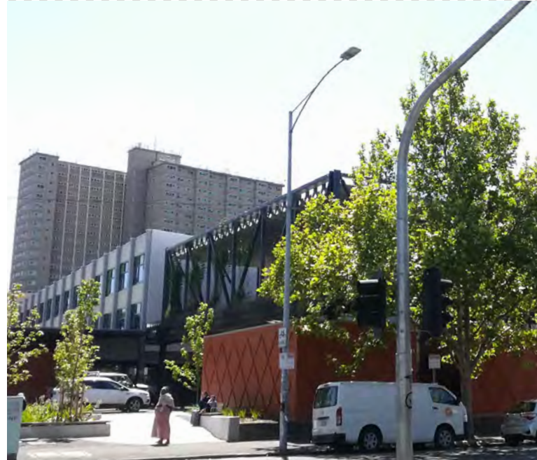
Figure 3.40 Primary school and public housing in Carlton
