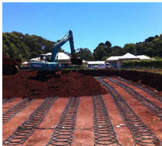
A large horizontal "slinky" system being backfilled as part of the extended research project.
