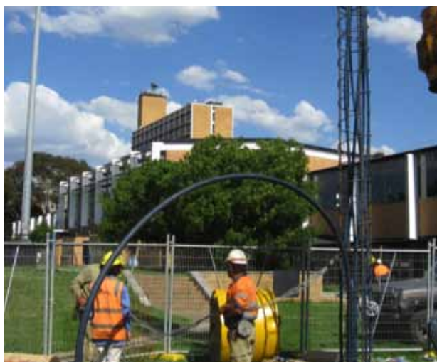
An energy pile being installed at the Beaurepaire Centre.
